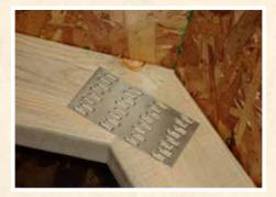
Metal Truss Plates Provides superior strength versus wooden gussets.
