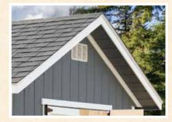
Smartside Soffit and Frieze Board
